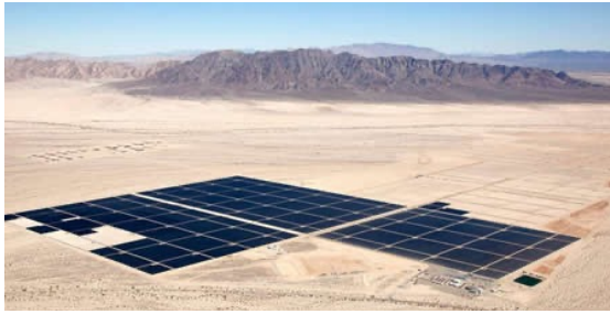
Figure 10: Solar Farms, Harbert Management Corporation 17
